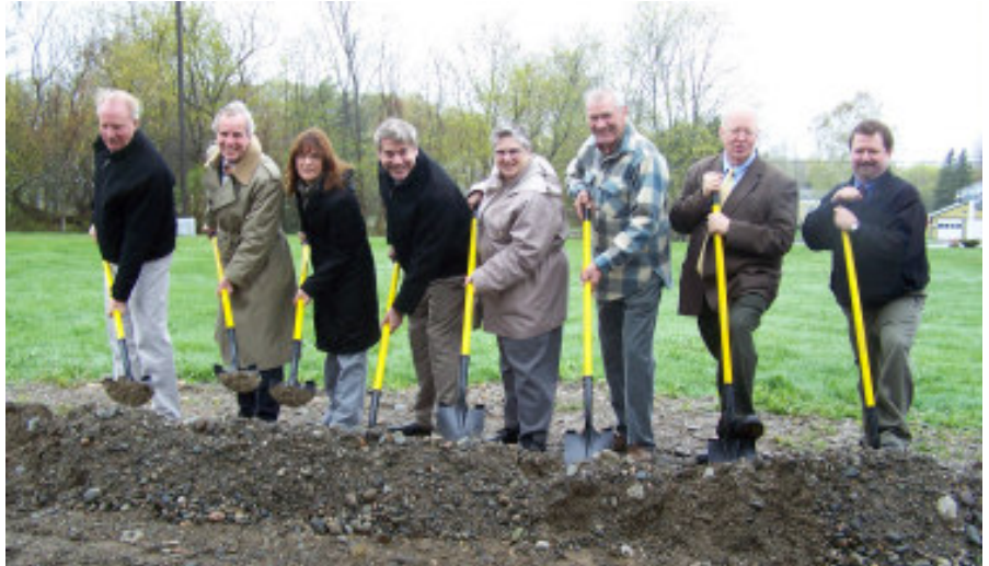
L-to R; Taking part in the groundbreaking ceremony was Dr. Christopher Hayward, CEO Michael Lally, Director of Practice Management Cammi Deschene, Dr. Mike Kessler, Board Chair Linda Gralenski, Building and Grounds Committee Chair Lawrence Clark, Dr. Bob Chagrasulis, and Family Nurse Practitioner Christopher Scalabrin.
